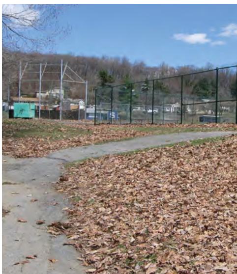
Tennis Court access does not meet ADA criteria
