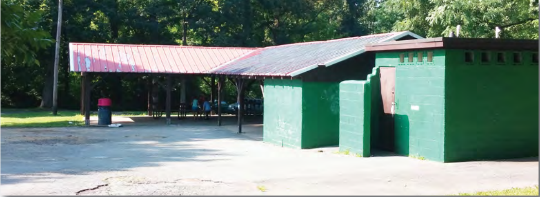
Laubach Park Pavilion & Rest Room Building
