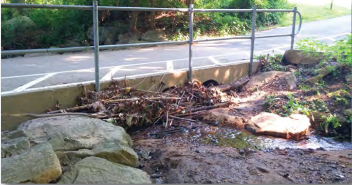
Laubach Park Pond Overflow Pipe
