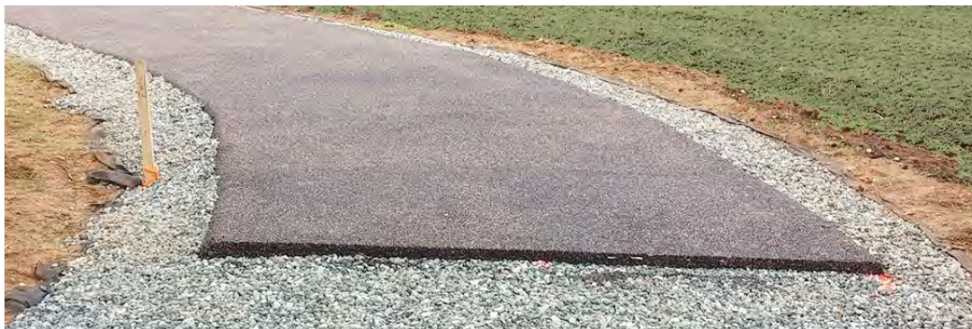
Lindberg Parks new Flexible Pervious Trail during install - 2015
