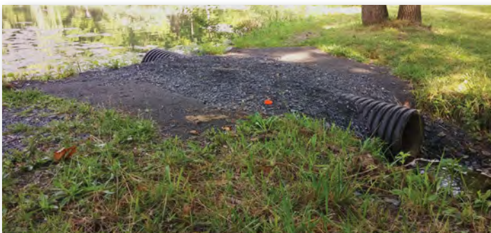
Laubach Park Pond Overflow Pipe
