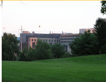
The Comprehensive Plan proposes new land use overlays allowing the Township to better manage growth at the Lehigh Valley Health Network Cedar Crest Campus Location.
