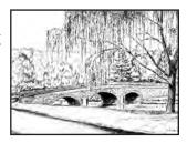
two surviving triple stone arch bridges that span the Little Lehigh River. The bridge, which is over 164 feet long, is constructed of cut and shaped stones; the bridge walls were recapped and railings were added in 1963.
