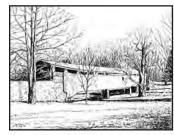
Lehigh Parkway (originally part of Salisbury Township,) the bridge is an example of a Burr-Truss type bridge, which utilizes an arch to help support the trusses, arranged triangularly on the bridge's sides.
